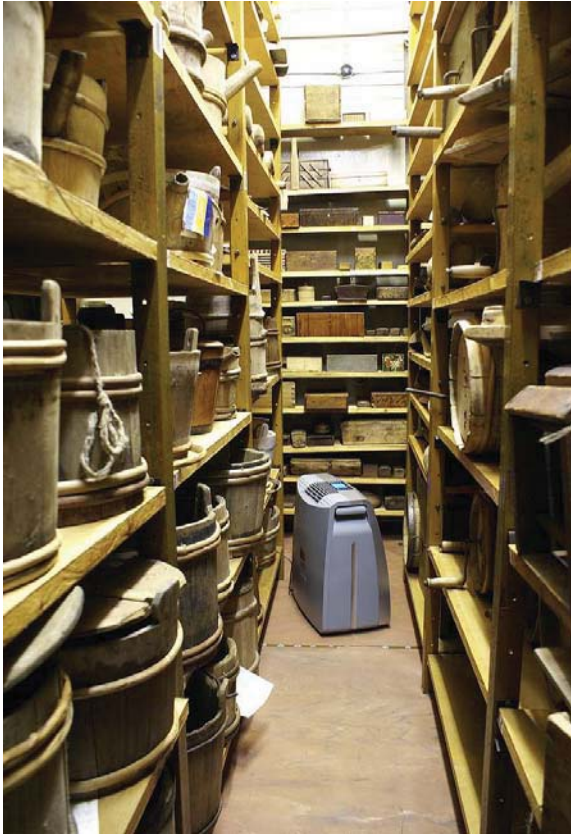
Photo 9: Use of dehumidifier to clean the air at the store room with mould problem.
