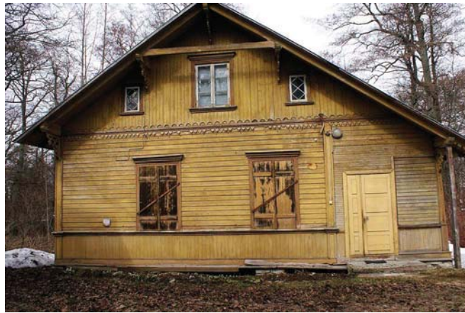
Figure 26: 1st depository facility of EOAM
