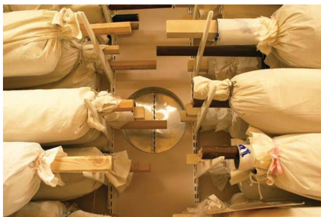
Figure 57: Holes in the wall for the anti-fire system.
