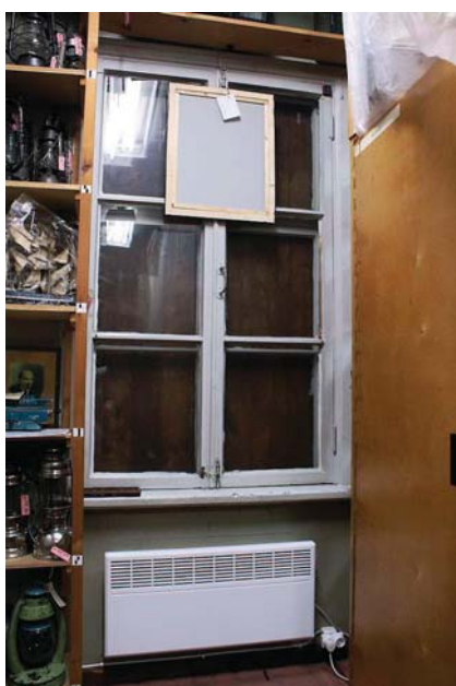
Figure 30: Use of radiators.
