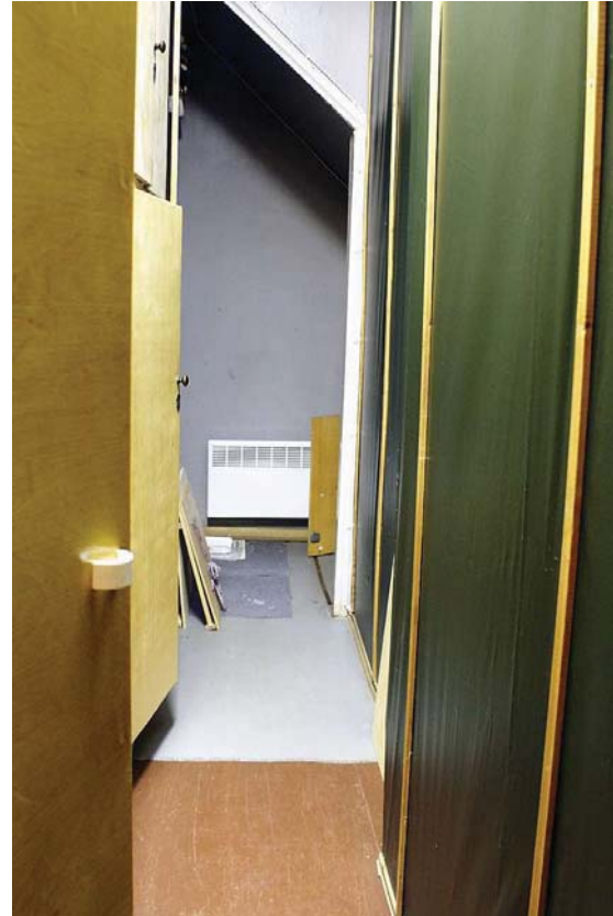
Photo 10: Narrow corridors that make difficult the access in the store rooms.
