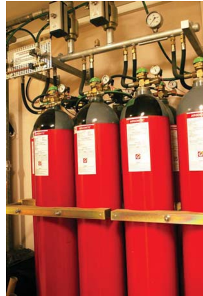
Figure 55: Anti-fire system Argonite.
