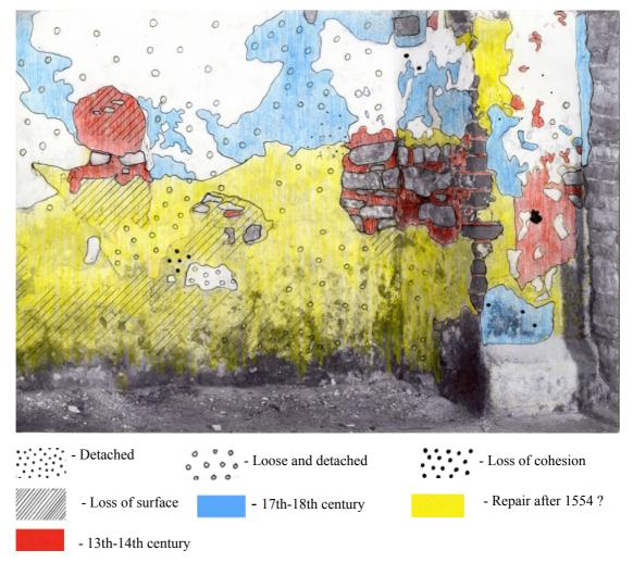
For my research, plaster from the Gothic construction period, which is the second building stage, was chosen as the reference for further tests. The first layer of the remaining plaster on the vaults and the walls, and also the painted decorations, belong to the 13<sup>th</sup>-14<sup>th</sup> century when the romanesque style church became gothic.<sup>20</sup>
