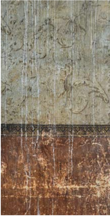
Figure 45. A wallpaper fragment from the Kabala manor showing monochromic dado, a narrow border and a wallpaper.
