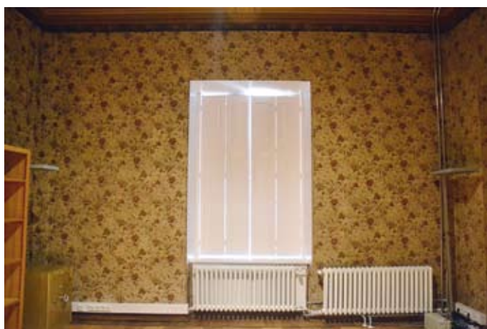
Figure 193. Final outcome of the restoration treatment.
