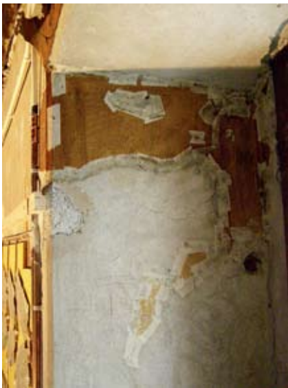
Figure 122. Edges of the wallpaper were consolidated with strips of Japanese tissue.
