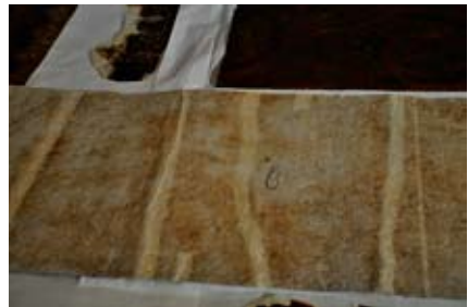
Figure 82. Removing heavy wallpaper from up downwards could result in numerous cracks and damaging the layer of paint.
