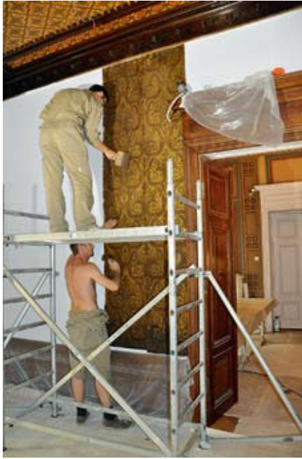
Figure 135. Each strip and segment was remounted to its original location.
