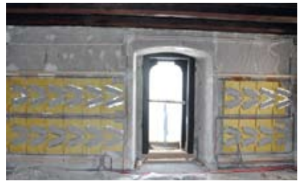
Figure 123. All the fragments were covered with a layer of a thin Manila hemp paper.
