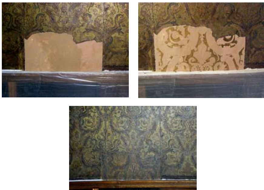
Figure 139. The reconstruction was painted in situ .
