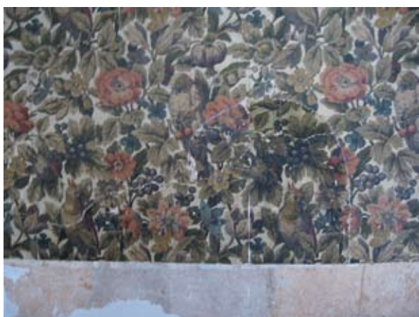
Figure 95. Large missing areas in the wallpaper were filled with fragments found behind the overdoors of the dining-room of the Puurmani manor.
