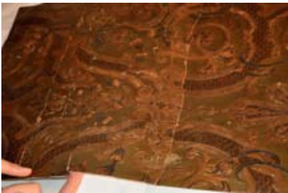
Figure 82. Removing heavy wallpaper from up downwards could result in numerous cracks and damaging the layer of paint.
