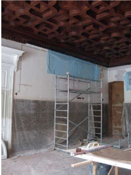
Figure 169. Dining-room of the Puurmani manor before restoration treatment.
