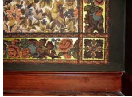
Figure 46. Plain paper integrated into tripartite decorative scheme in the dining-room of Puurmani manor.
