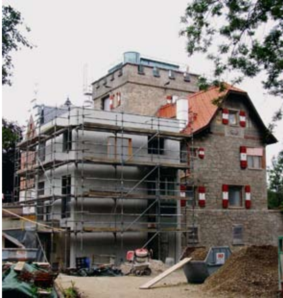
Figure 120. Freyschlössl during renovation and construction works in 2011.
