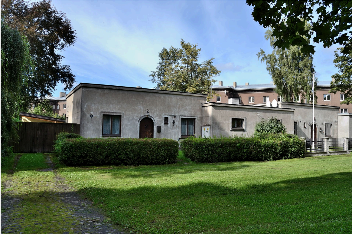
67. Maasika 4/6, Tallinn. foto- https://et.wikipedia.org/wiki/Maasika_t%C3%A4he_tn_39/Lootuse_pst._107_eramuga_v%C3%A4ga_sarnased_uksed
